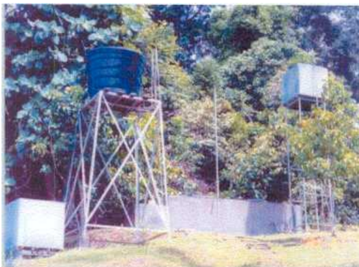
Plate No 12: Water tank to store water pumped from Danum River at the Danum Research Center
