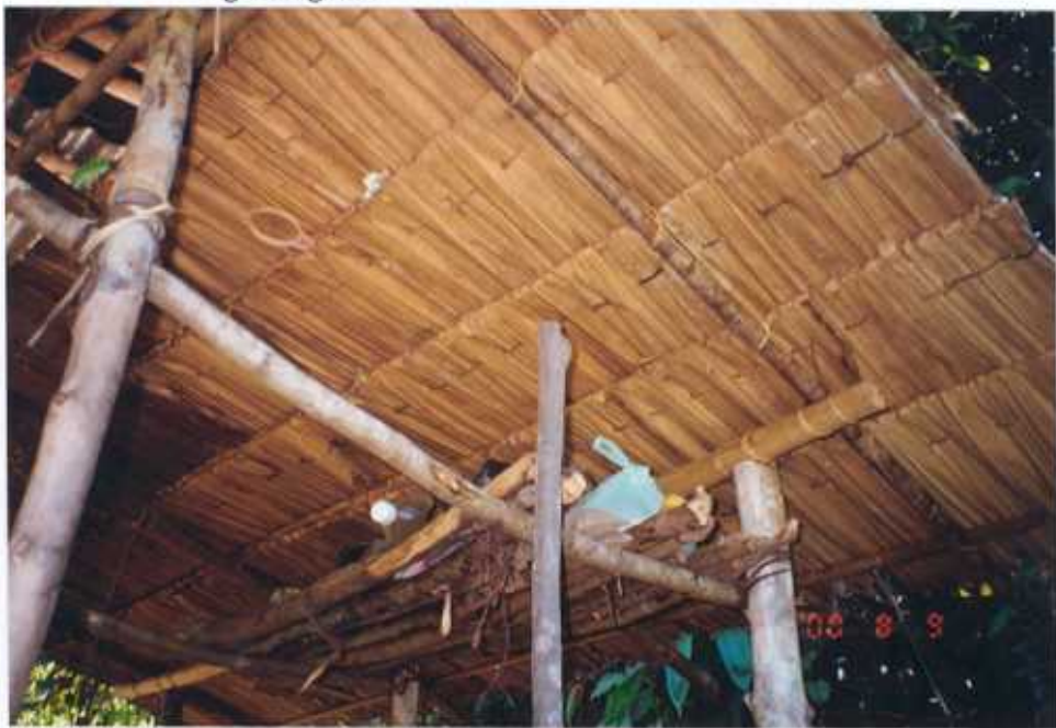
Fig. 50 : Roof tatching made from 'Nipah' leaves
