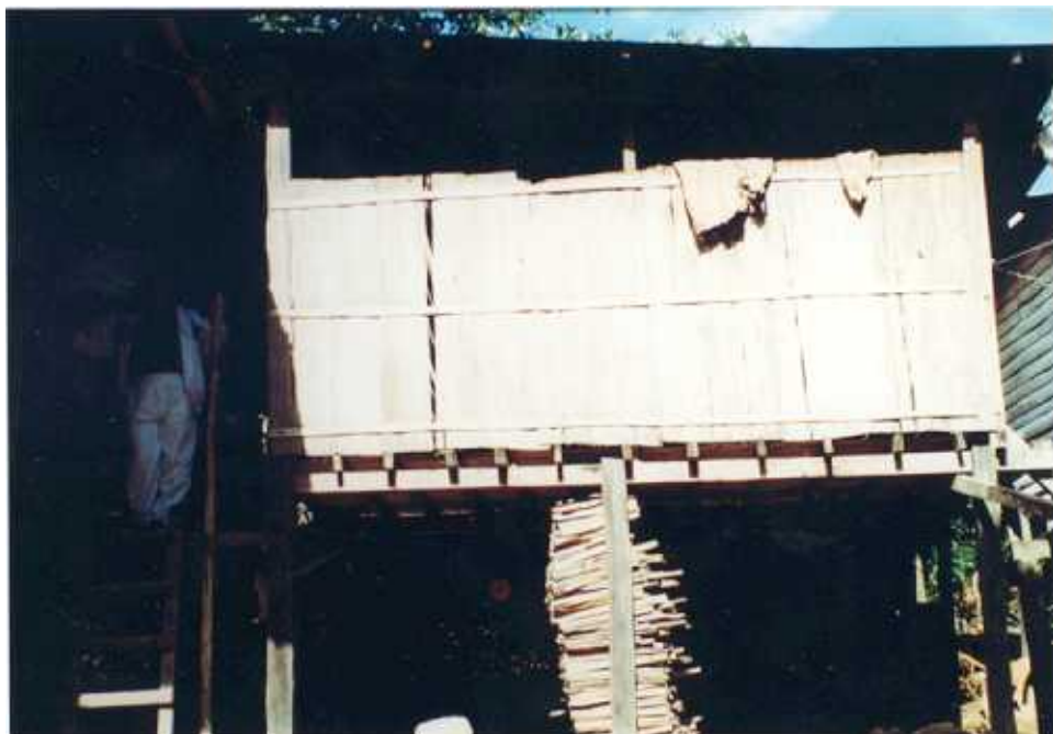
Fig. 48 : The Murut Tanggala's house wall is made from tree bark
